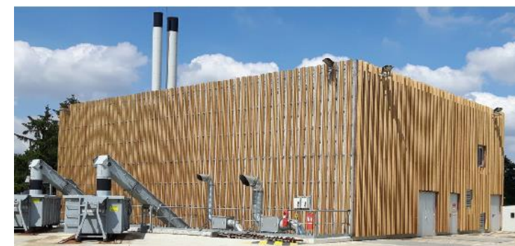
Chaufferie biomasse de Saint-Germain-en-Laye
